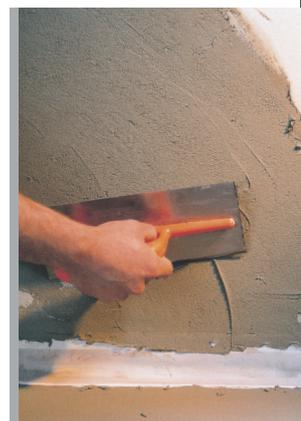
**Aggregates :** Aggregates used in the mortar / concrete should be well graded and thoroughly washed. Sand particles sizes should correspond to the thickness of mortar to be applied.
